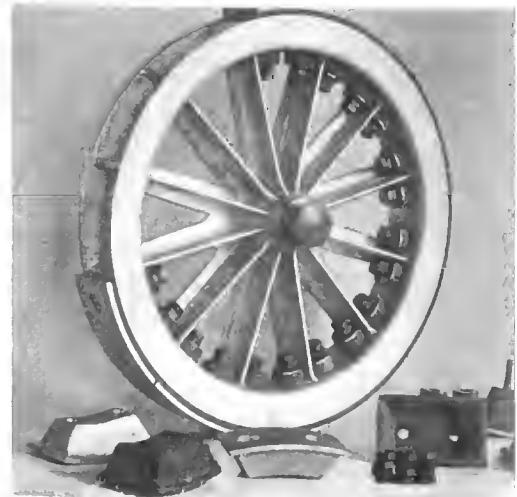
View of Lea Wheel and Sections of the Tire.
